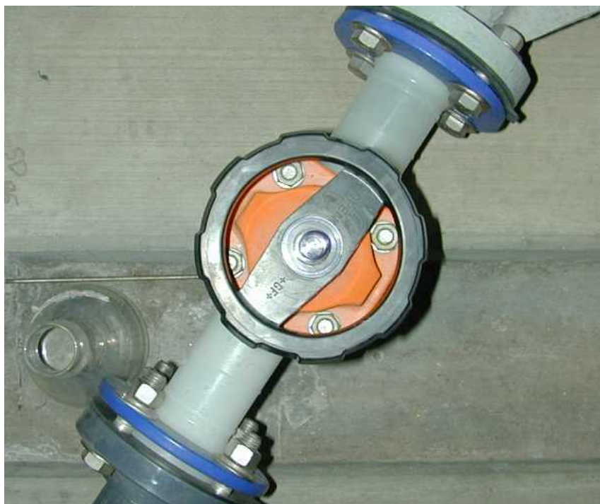
FIGURE 9. The HALAR tank drain valve, TVdr.
