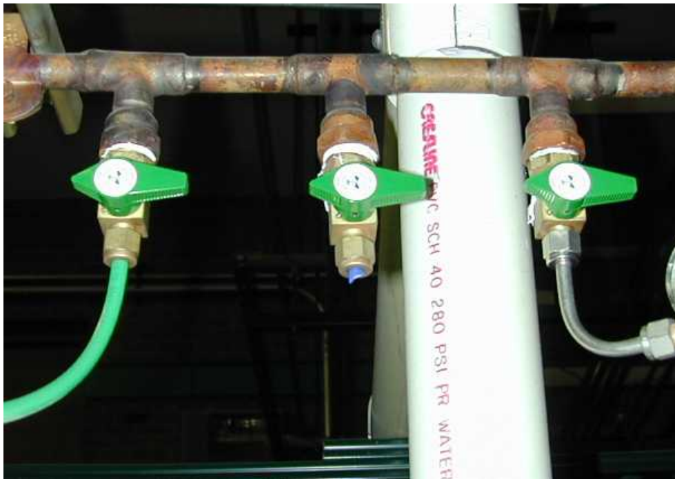
FIGURE 12. Pneumatic pump gas lines.
